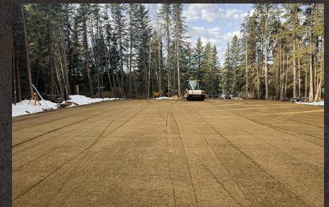
Compacting the top layer of Tough Cell®.
