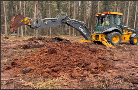
Site logging, clearing and preparation.
