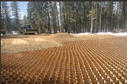
Filling first layer with gravel.
