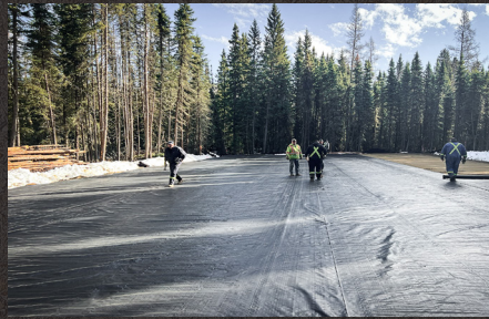
Laying geotextile.
