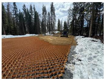
development practices. The technology allows for the use of recycled and locally sourced materials, reducing the need for transported aggregate and expediting installation processes.
