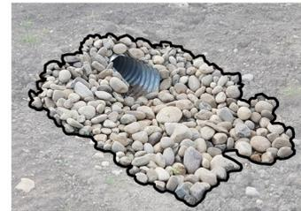
A minimum 500 mm (20 inch) diameter, **new** Corrugated Steel Pipe culvert is required
