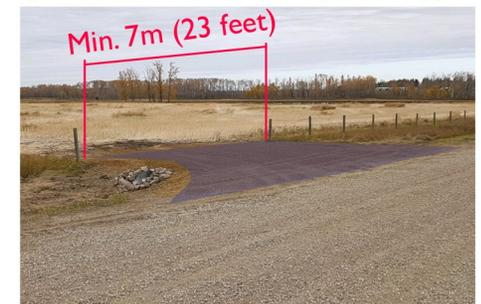
A minimum 3 Horizontal to 1 Vertical rate of slope is required on either side of the approach
