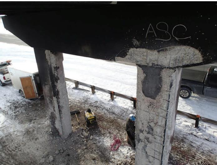
Fire Damaged pier after some heat damaged concrete has been removed
